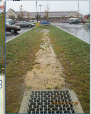
Commercial: Parking Island Filtration / Infiltration
