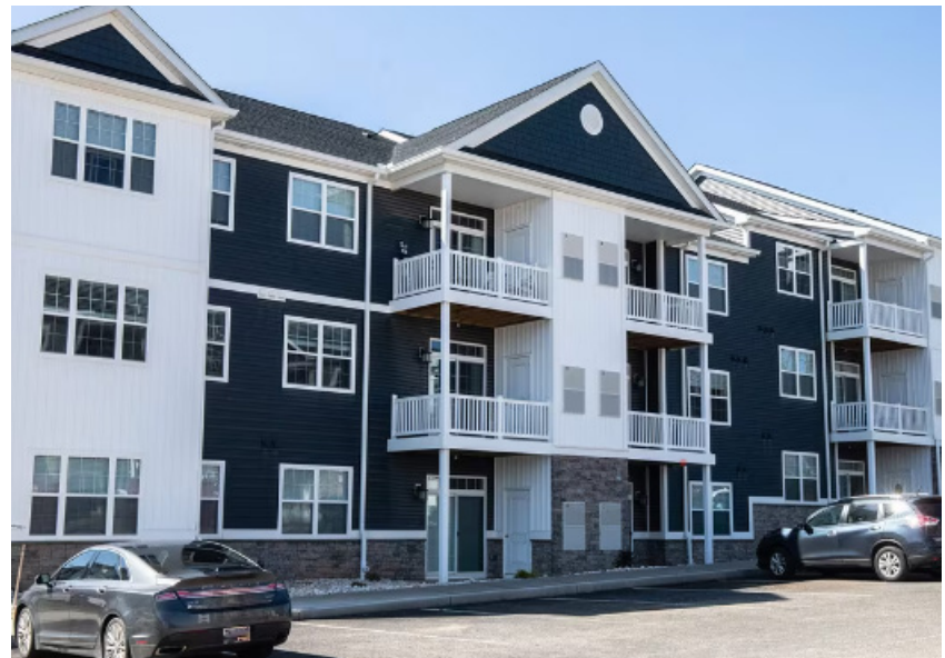
Abbey Place Multifamily Complex Image Source: https://www.apartments.com/abbey-place-westminster-md/7x5582y/
