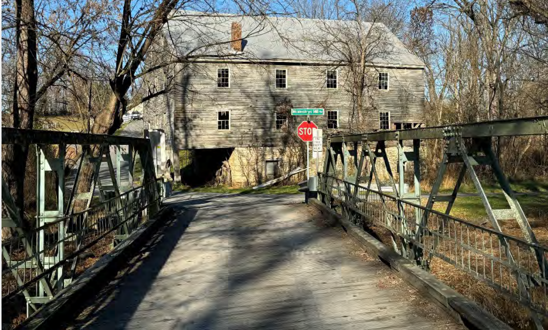
(Photo: Pearre Road Bridge over Sams Creek)
