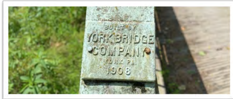
(Photo: Pearre Road Bridge over Sams Creek)
