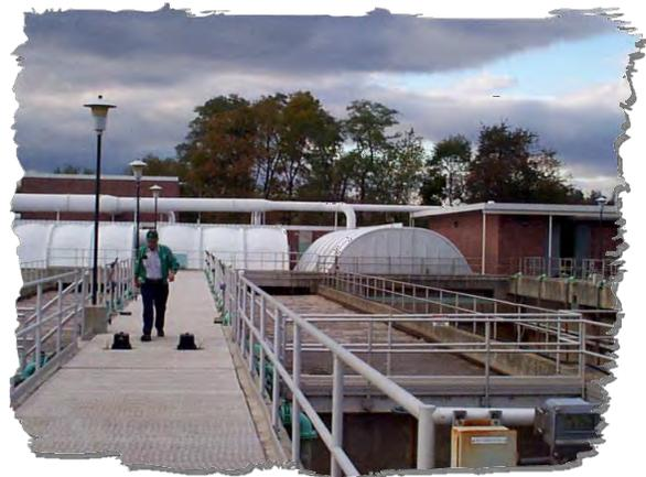
The upgrade from biological nutrient removal (BNR) to enhanced nutrient removal (ENR) technology does not include plant expansion. There are, however, future plans to expand the plant from 5.0 mgd to 6.5 mgd, if needed. Analysis in this section assumes that the plant capacity expansion to 6.5 mgd will not be implemented within the next 10 years.
