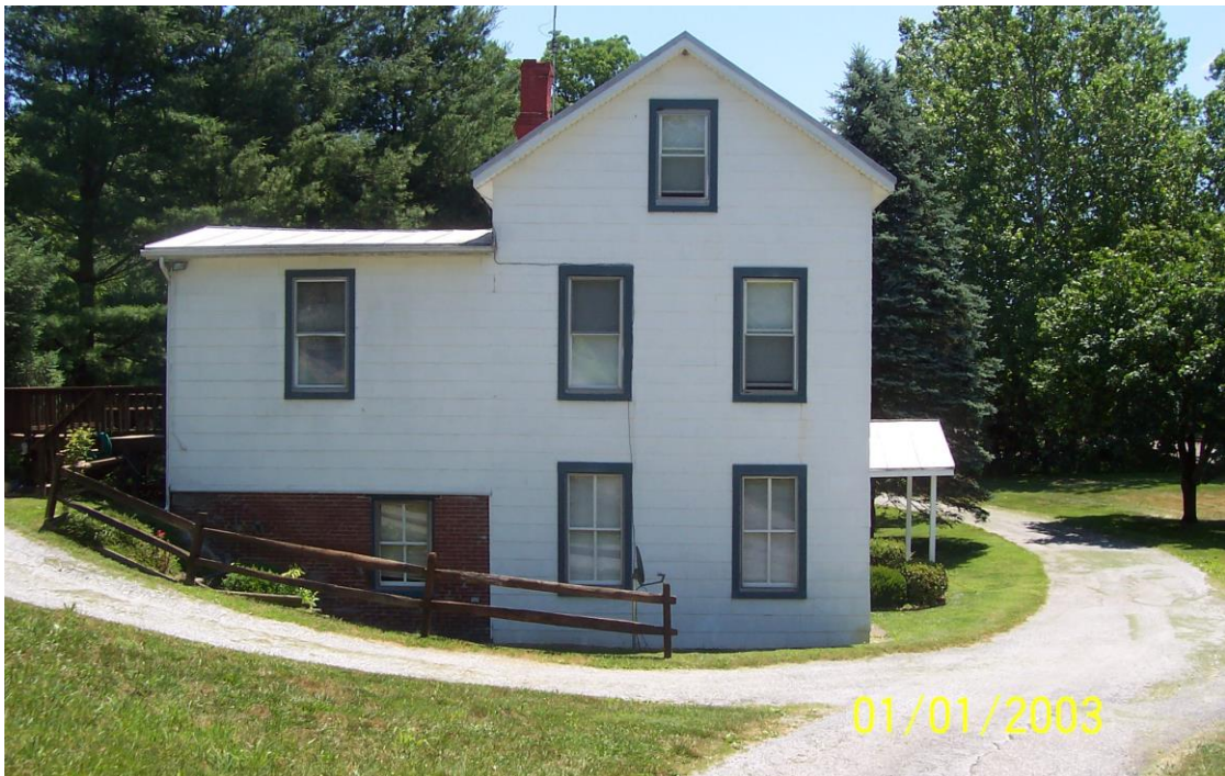
LEFT(NORTHWEST) SIDE VIEW – 6/15/11
