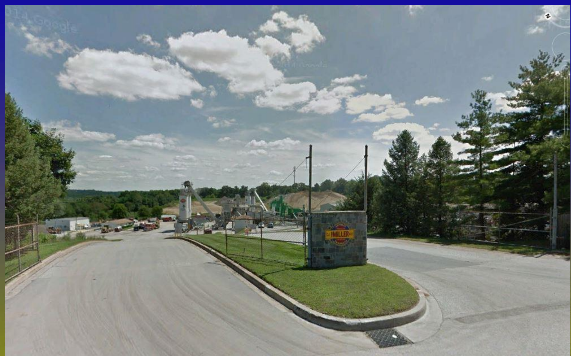
Finksburg Asphalt Plant
