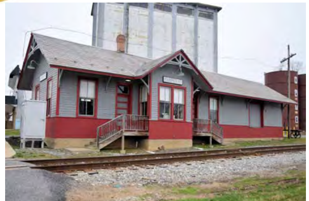
Hampstead, MD train station now
