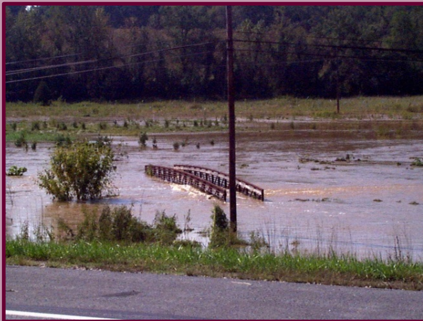
Little Pipe Creek Park Bridge
