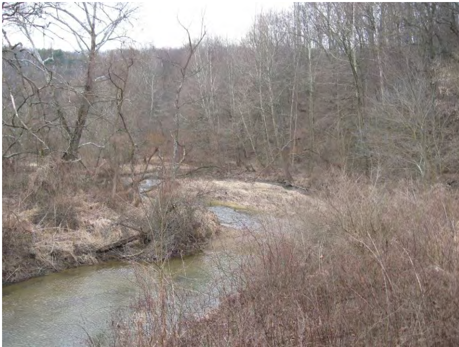
Photo 2 – View upstream from Saw Mill Road at dam site.
