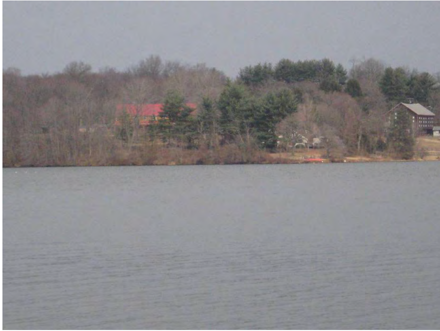
Photo 7 – Historical structure on east side of reservoir.
