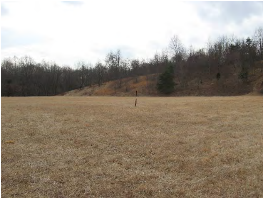
Photo 2 – Downstream view of emergency spillway.
