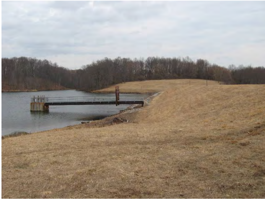
Photo 3 – Overview of upstream slope of dam.
