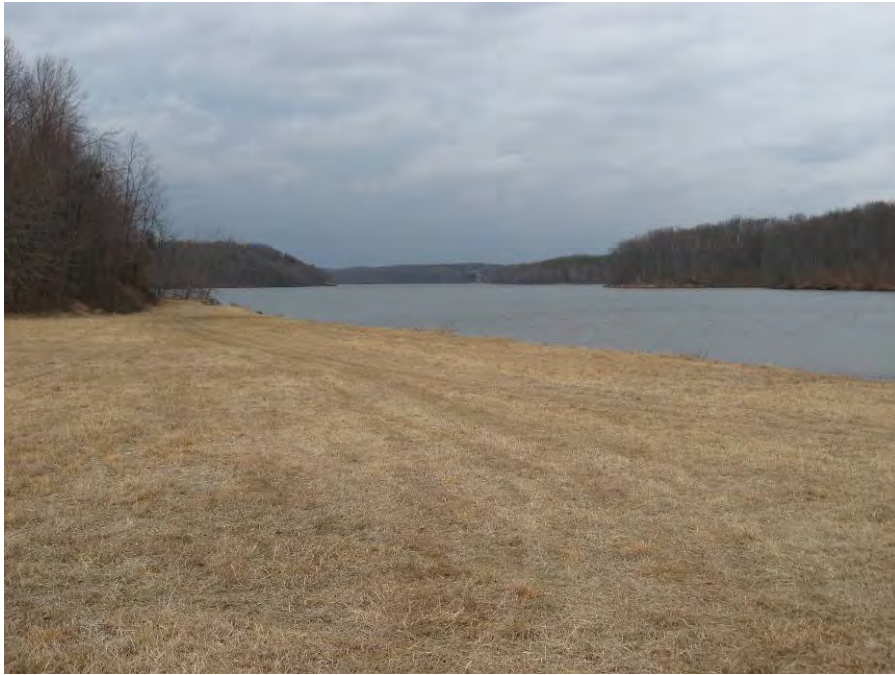
Photo 1 – View upstream from emergency spillway.
