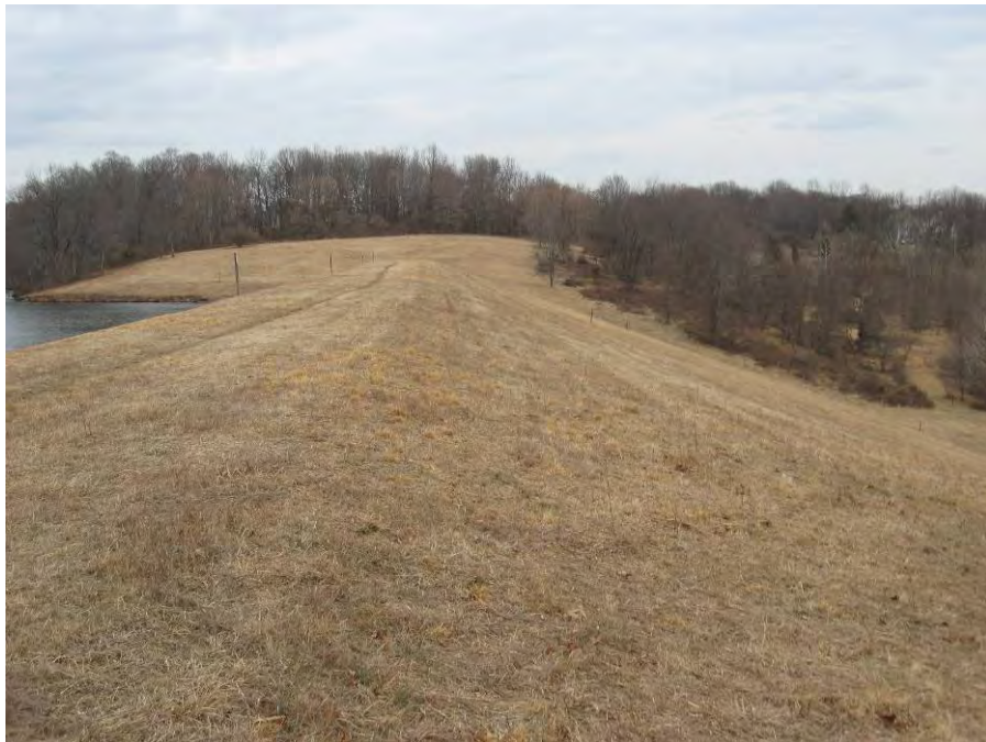
Photo 4 – Overview of downstream slope of dam.
