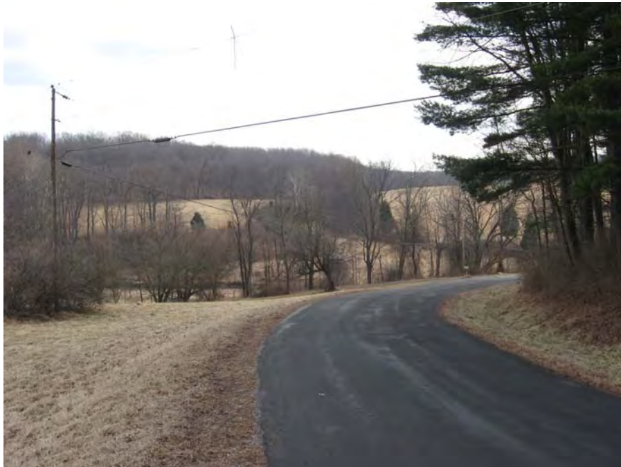
Photo 8 – View across valley to right abutment.
