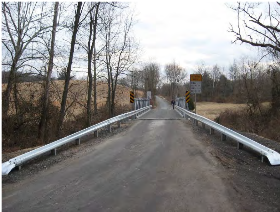
Photo 1 – View across bridge at Saw Mill Road at dam site.
