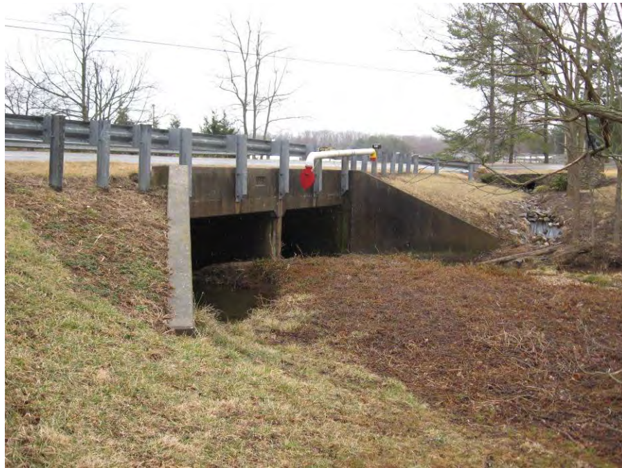
Photo 3 – View of road culvert at Runkles Road.
