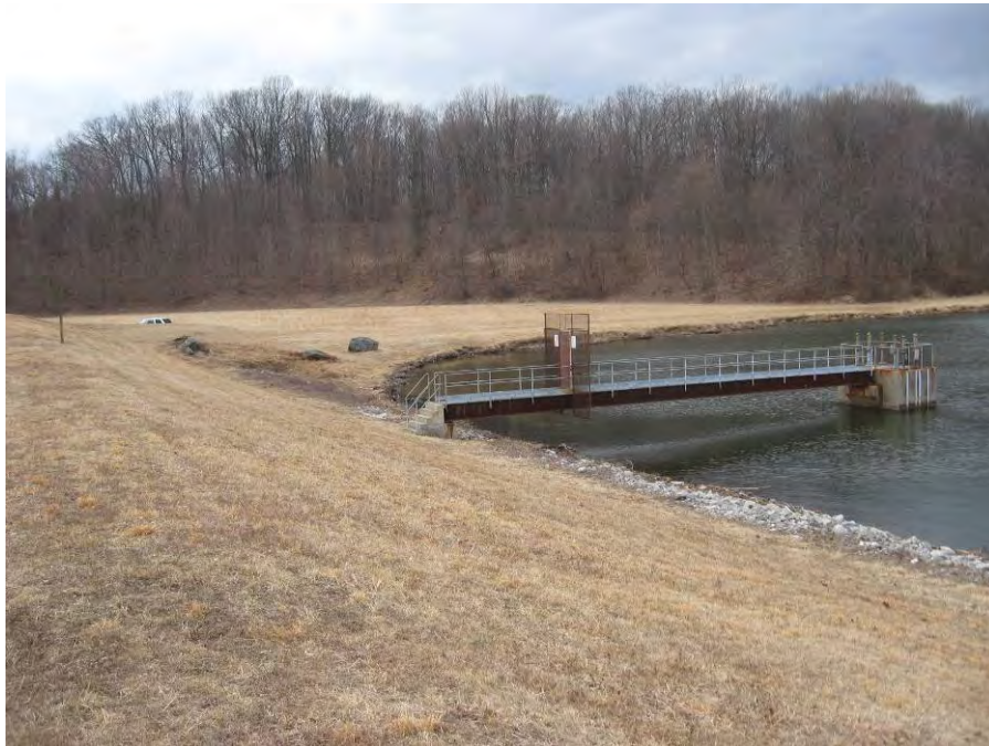
Photo 6 – Intake structure and pedestrian bridge.
