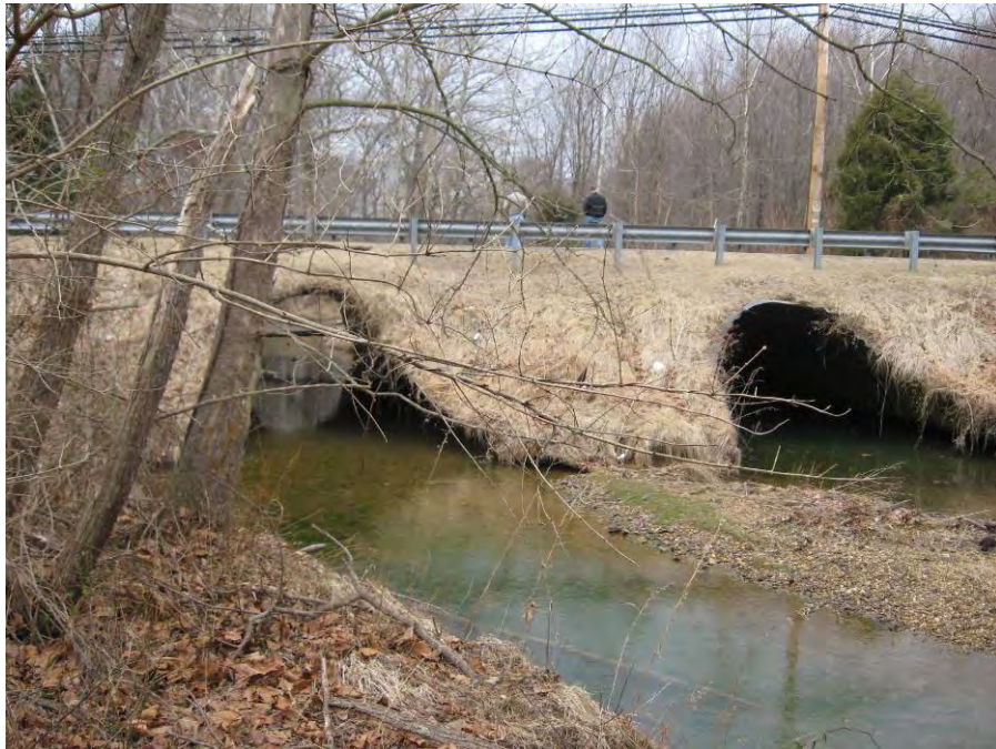
Photo 8 – View of road culvert at White Rock Road.
