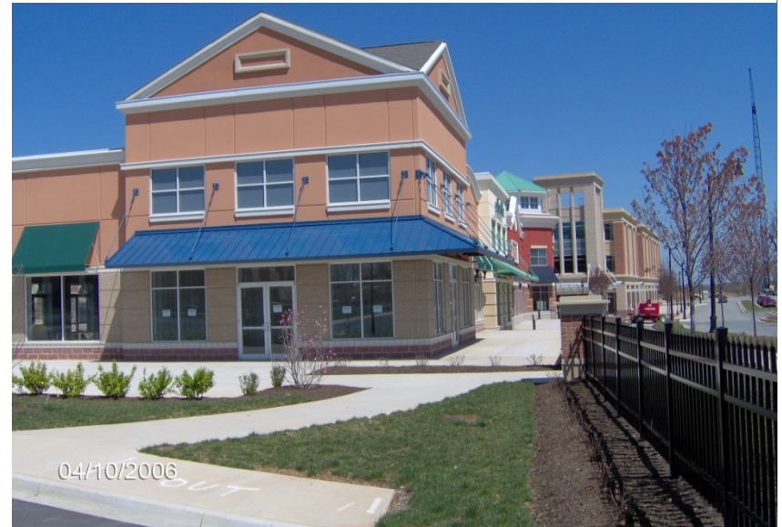
(Below) Even the illusion of a second story helps to define space.
