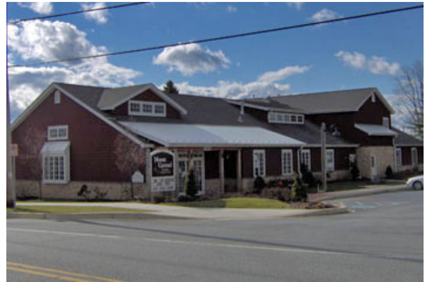
(Below) This veterinarian clinic in rural Maryland uses color, material, form and scale to fit in with the surrounding area.
