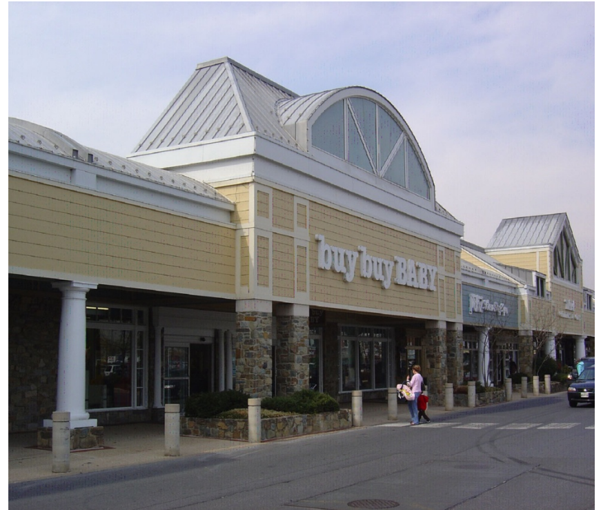
(Above) This shopping center demonstrates the application of universal design features, using a flush curb edge and bollards to create a safe and barrier-free pedestrian way.
