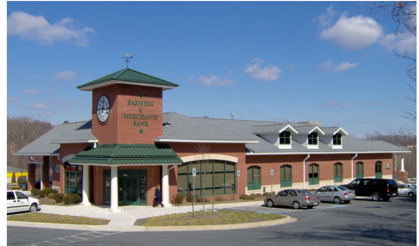
(Above) The varied roofline, corner tower, and gabled roof with dormers on this bank help to reduce the bulk of the building and break up the mass of surfaces.
