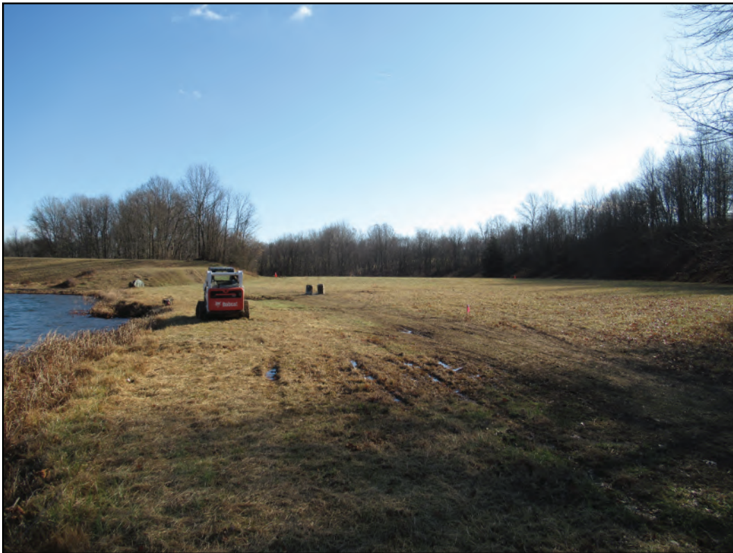
Figure 6-9. Emergency Spillway, Facing South
