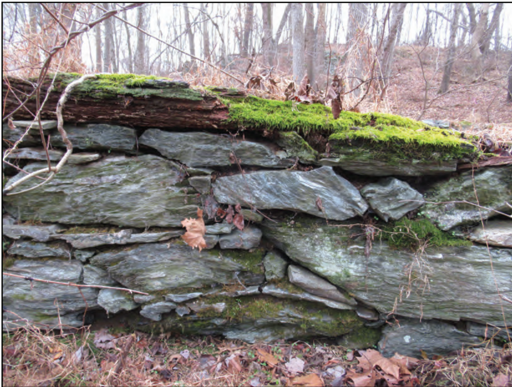
Figure 6-28. 18CR293, Feature 2 Stonework and Timber Sill Plate Detail, Facing South
