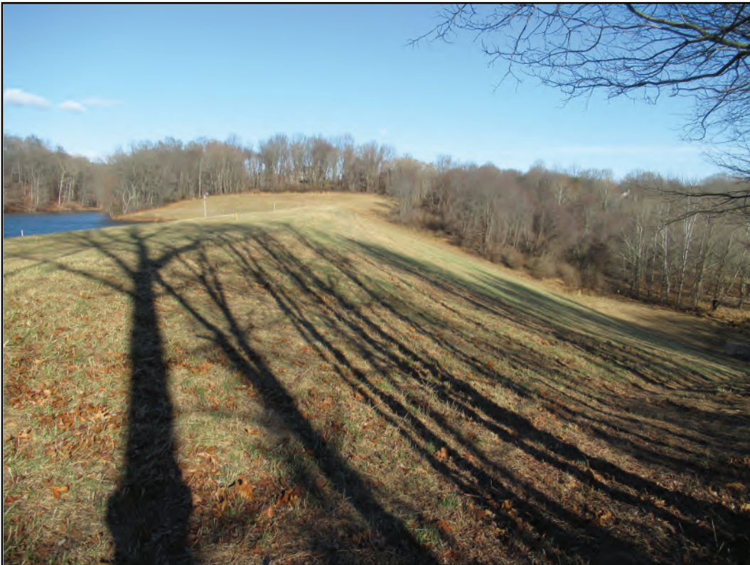
Figure 6-8. Piney Run Dam, Facing East
