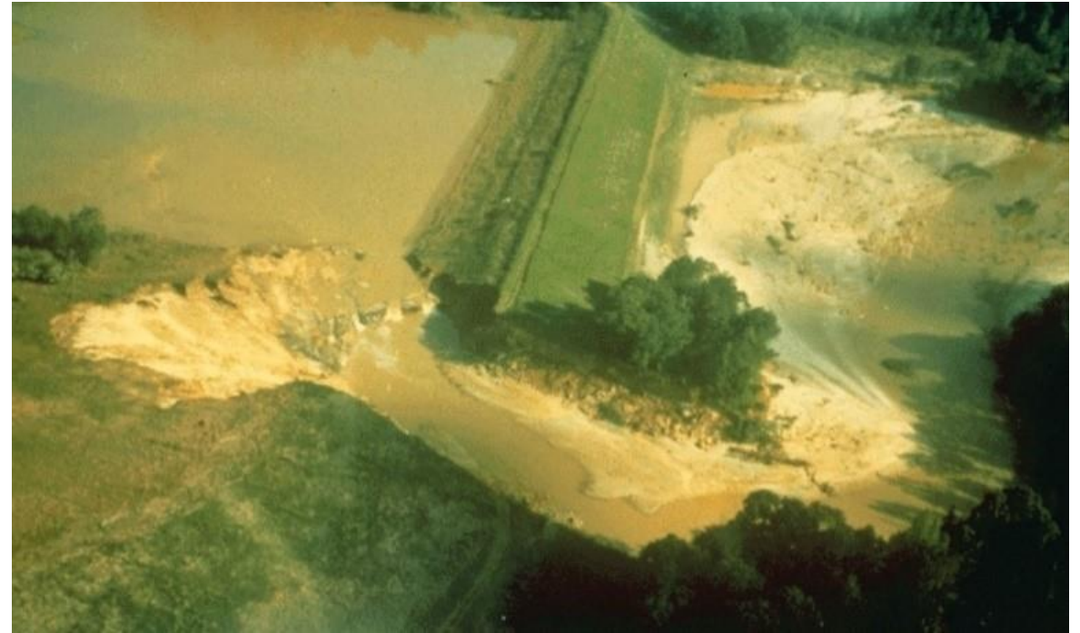
Black Creek Site 53 (MS) failure from spillway erosion in 1983 (courtesy: NRCS)
