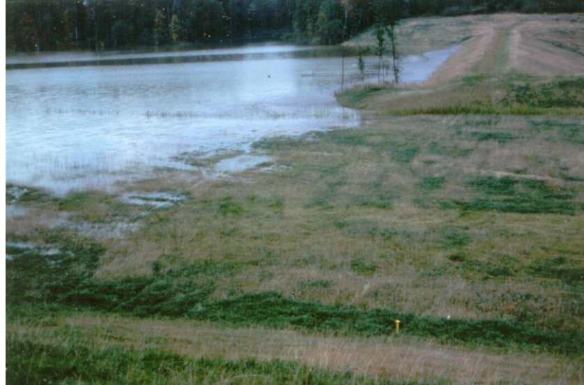
Piney Run auxiliary spillway during Hurricane Eloise (1975)
