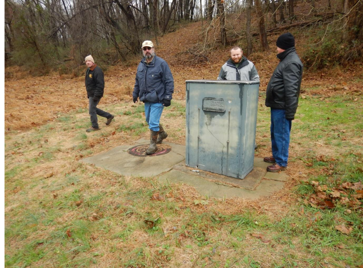
Inspection of Piney Run water supply conduit rate control vault.
