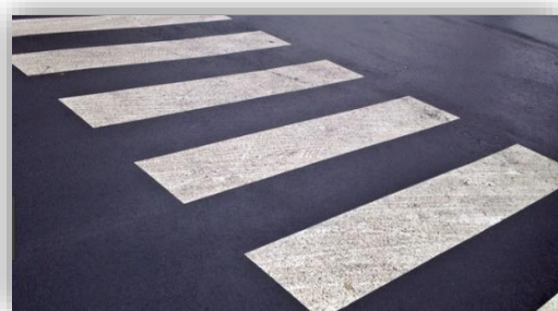
Figure 6-3: Block pattern crosswalk
